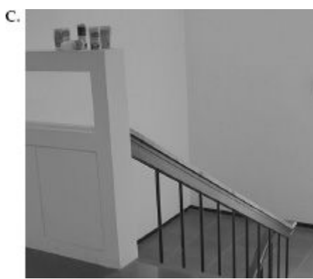
FIGURE 1.5. Accidental Affordances Can Become Strong Signifiers. This wall, at the Industrial Design department of KAIST, in Korea, provides an anti-affordance, preventing people from falling down the stair shaft. Its top is flat, an accidental by-product of the design. But flat surfaces afford support, and as soon as one person discovers it can be used to dispose of empty drink containers, the discarded container becomes a signifier, telling others that it is permissible to discard their items there. (Photographs by the author.)
